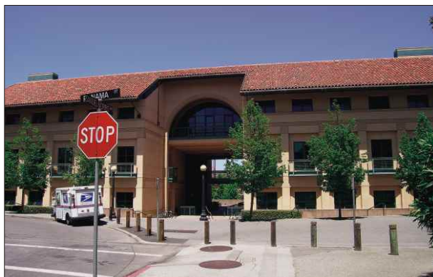
The Green Earth Sciences Building
